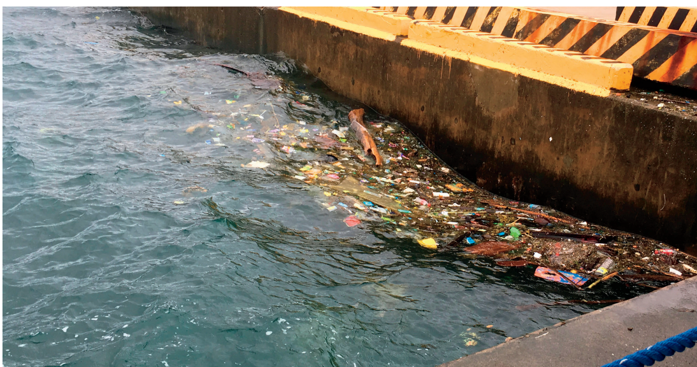
Observed leakage of waste including plastics in a port
